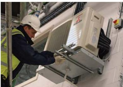
A total of 132 ceiling ducted indoor units from MHI's KX6 range are being installed throughout the Hampton Hilton Hotel in a range of capacities. The majority of guest rooms have FDUM22KXE6 low-noise units with 2.2kW cooling and 2.5kW heating capacities, while the open plan breakfast area, for
